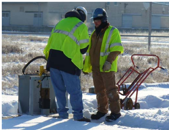
Figure 6. Concrete Core Sampling Team.
