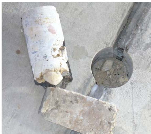
Figure 7. Core at Expansion Joint.
