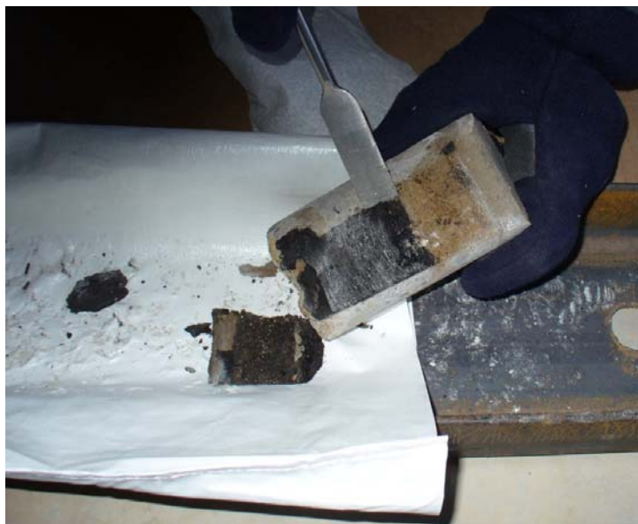
Figure 2-14 Removal of Expansion Joint Material (EJM)
