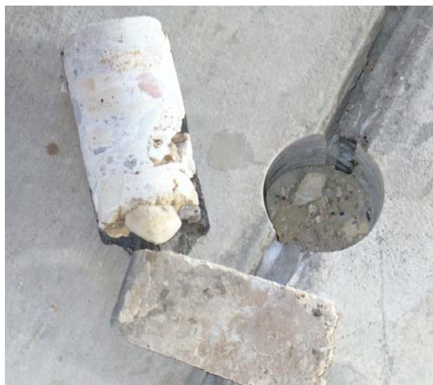
Figure 2-8 Core Taken at Expansion Joint
