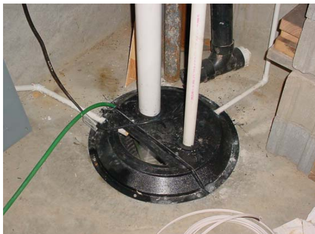
Figure 4-2. Passive sump mitigation system.
