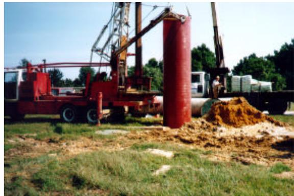
Figure 6. Fiberglass liner of the test well being lowered into place at CBD
