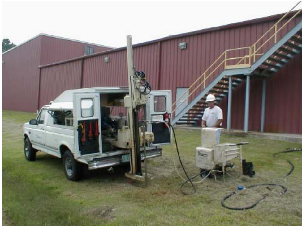
Figure 1.7 Direct Injection of Pure Edible Oil through Geoprobe® Rods Using a Grout Pump
