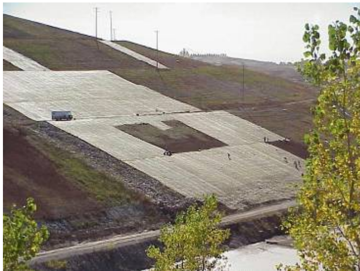
Figure 4-7. Final cover erosion control system. (Courtesy Kansas Department of Health and Environment)
