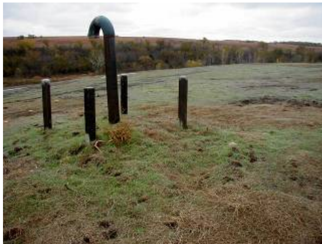
Figure 4-5. Landfill gas vent. (Courtesy Kansas Department of Health and Environment)
