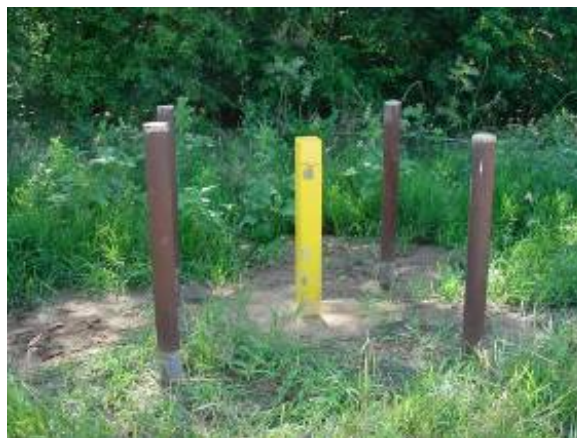
Figure 4-6. Groundwater monitoring well. (Courtesy Kansas Department of Health and Environment)
