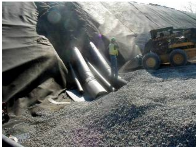
Figure 4-3. Leachate riser. (Courtesy Kansas Department of Health and Environment)
