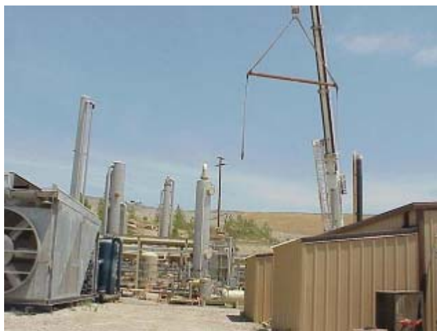
Figure 4-4. Landfill gas treatment plant. (Courtesy Kansas Department of Health and Environment)
