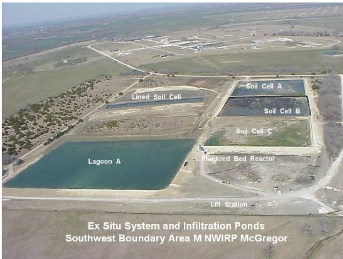
Figure A-36. FBR location at Area M.
