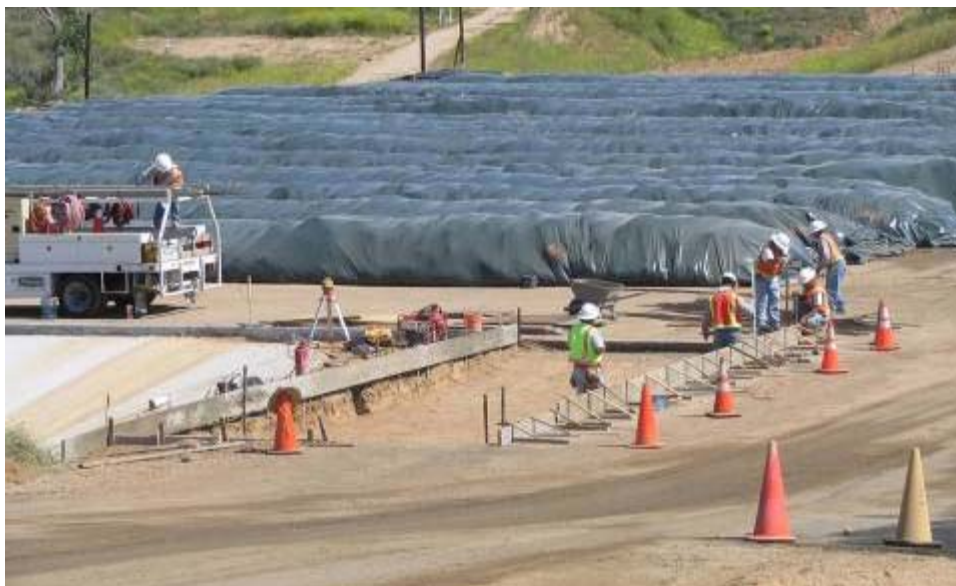
Figure 8-6. Staged Ag-Bags filled with soil. (Courtesy CDM Corp.)
