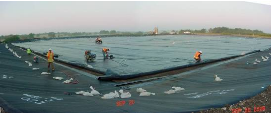
Figure A-39. Liner installation at Soil Cell C construction at Area M.
