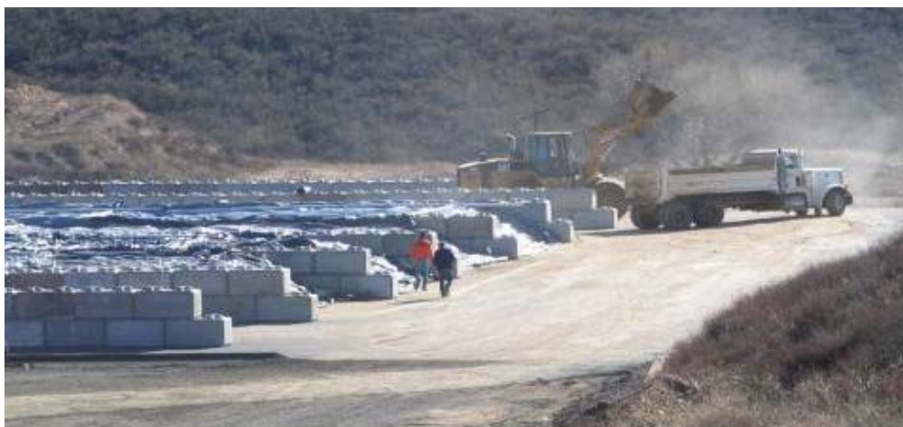
Figure 8-7. Cement-lined treatment cells. (Courtesy CDM Corp.)
