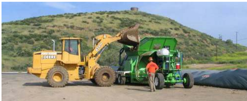
Figure 8-5. Ag-Bag being filled with soil. (Courtesy CDM Corp.)
