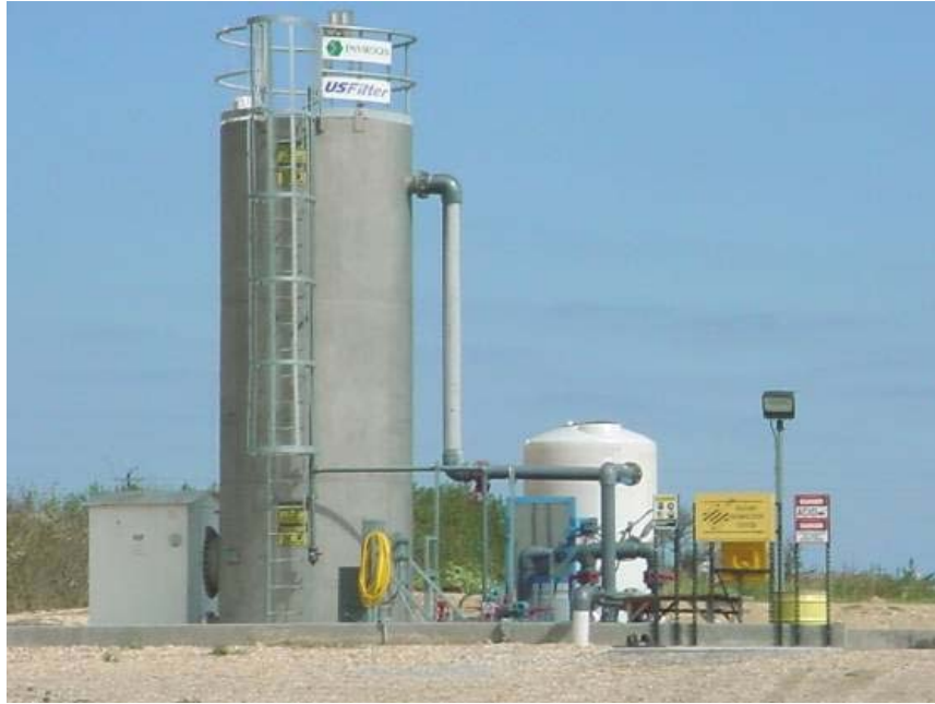
Figure A-37. FBR installed at Area M.
