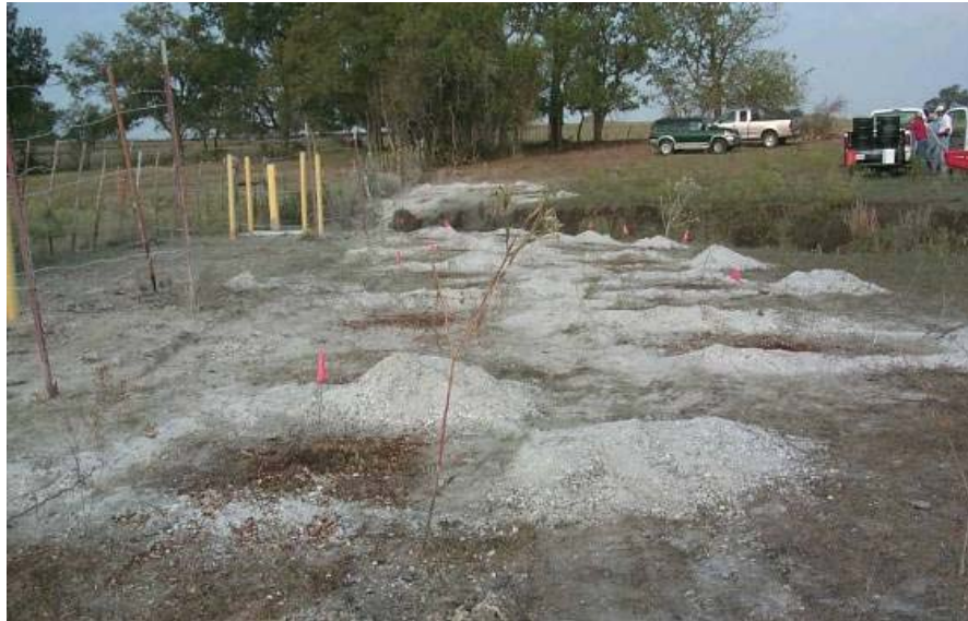
Figure A-34. Bioboring row after completion.
