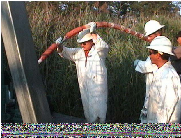
Figure 19. Preparation and installation of Multilevel Monitoring System (MLMS) at wetland study site: (clockwise from upper left) coiled 7-chamber polyethylene tubing, preparation of MLMS with sand packers and bentonite packers, drilling of borehole with vibratory rig, and insertion of MLMS down borehole casing. Precision Sampling, Inc. photos
