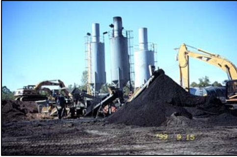
Figure 7-1. Ex-Situ Treatment at ACW
