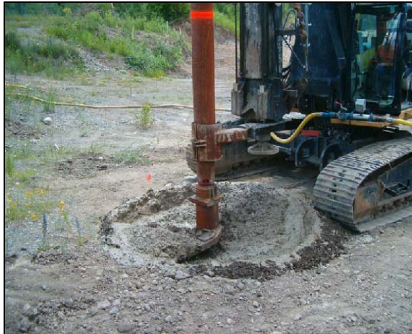
Figure 7-7. In-Situ Soil Mixing at MGP Site
