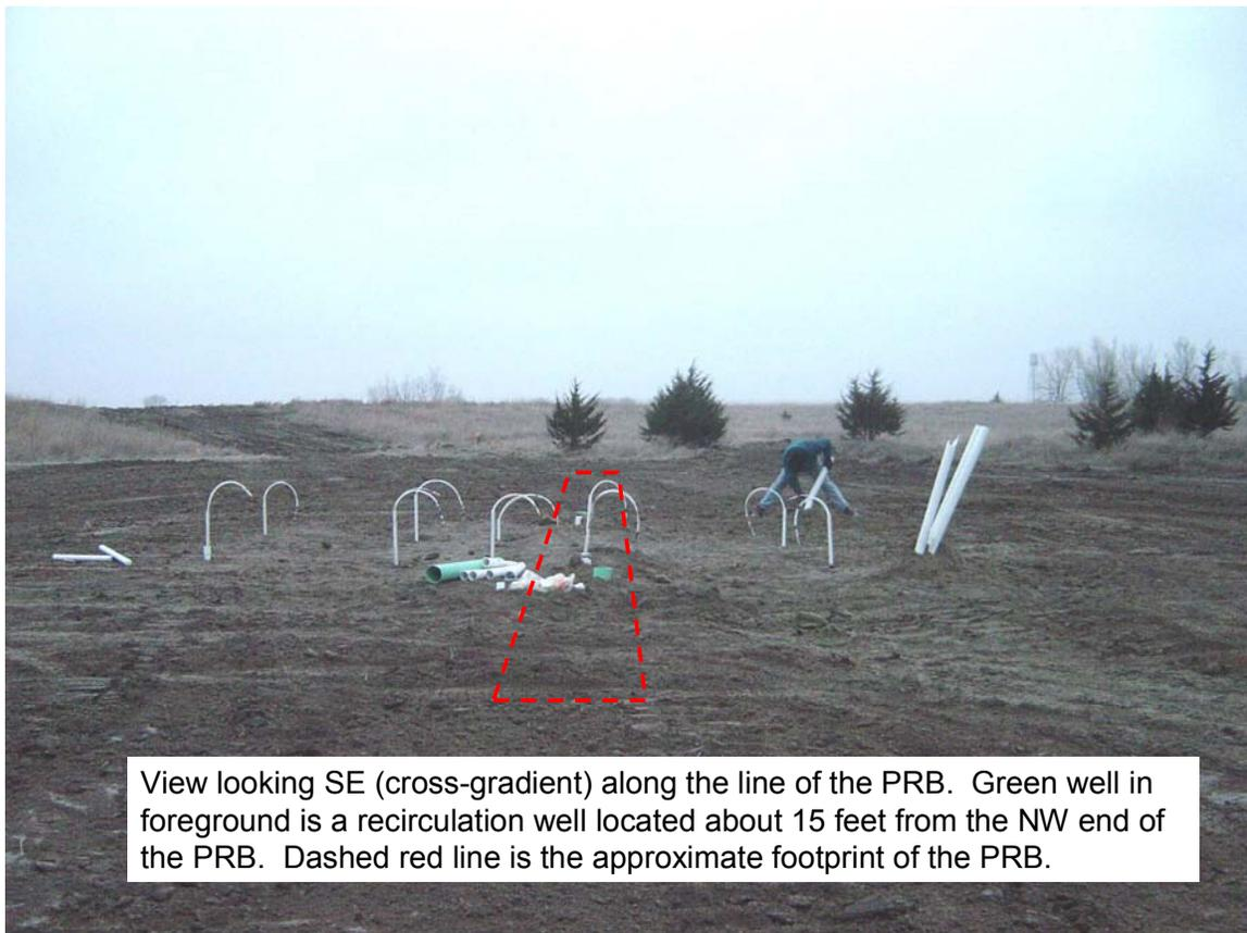
View looking SE (cross-gradient) along the line of the PRB. Green well in foreground is a recirculation well located about 15 feet from the NW end of the PRB. Dashed red line is the approximate footprint of the PRB.
