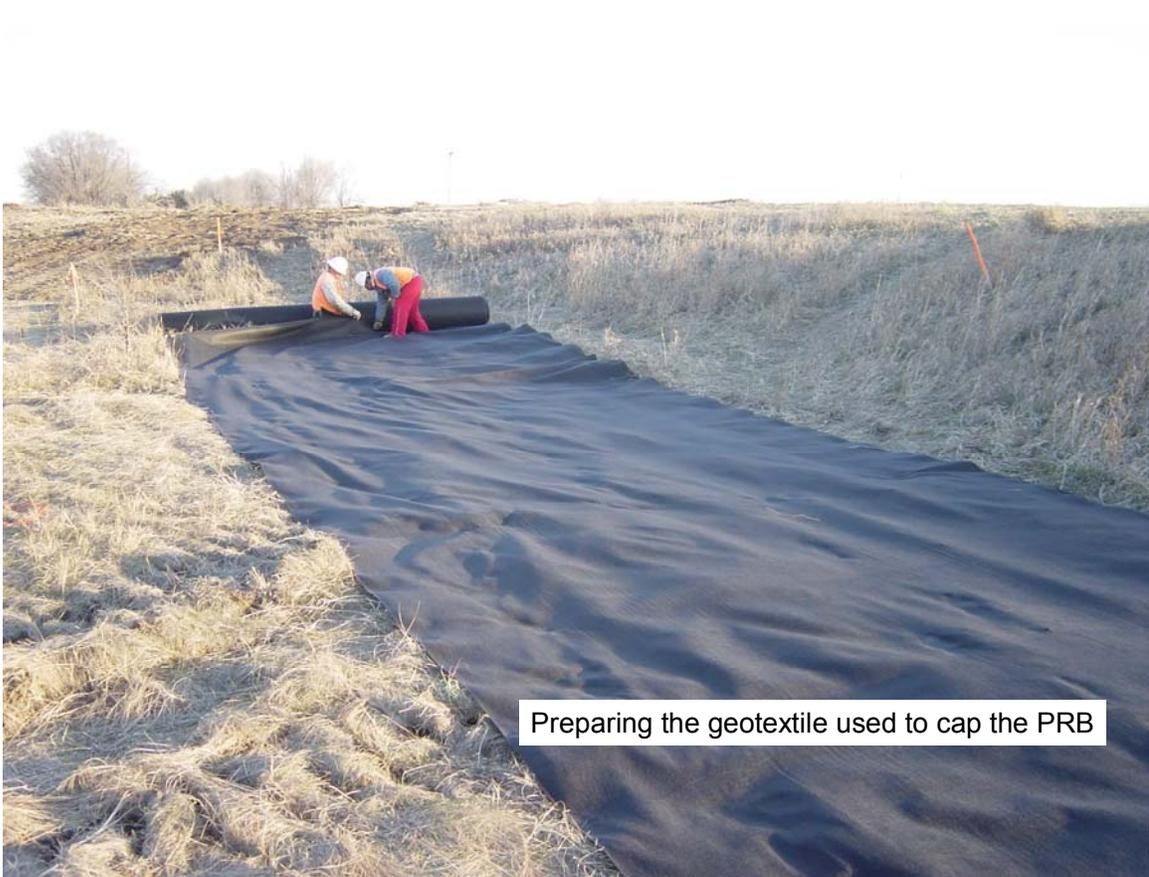
Preparing the geotextile used to cap the PRB
