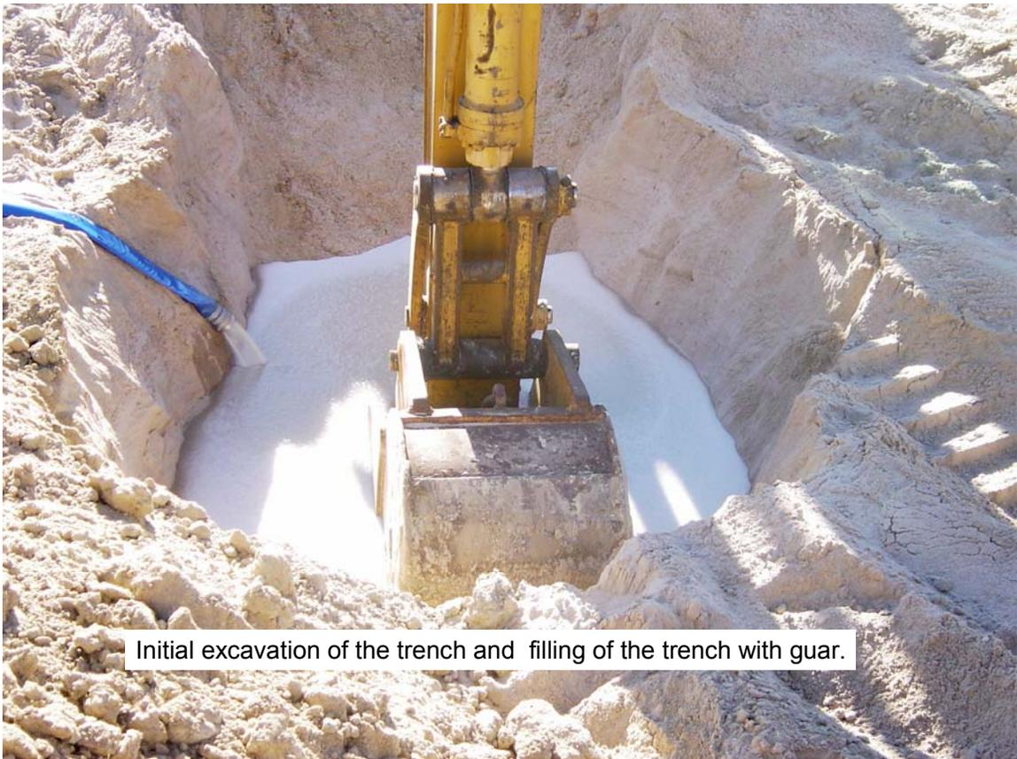
Initial excavation of the trench and filling of the trench with guar.
