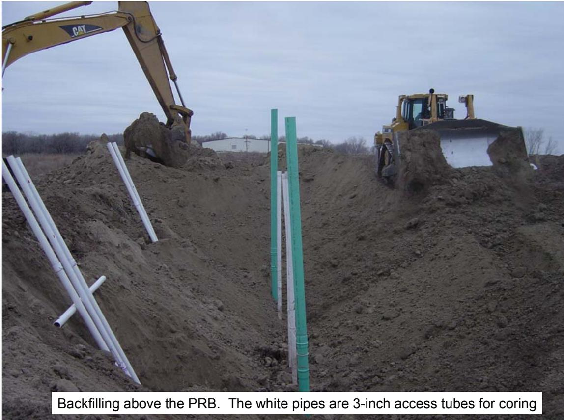
Backfilling above the PRB. The white pipes are 3-inch access tubes for coring
