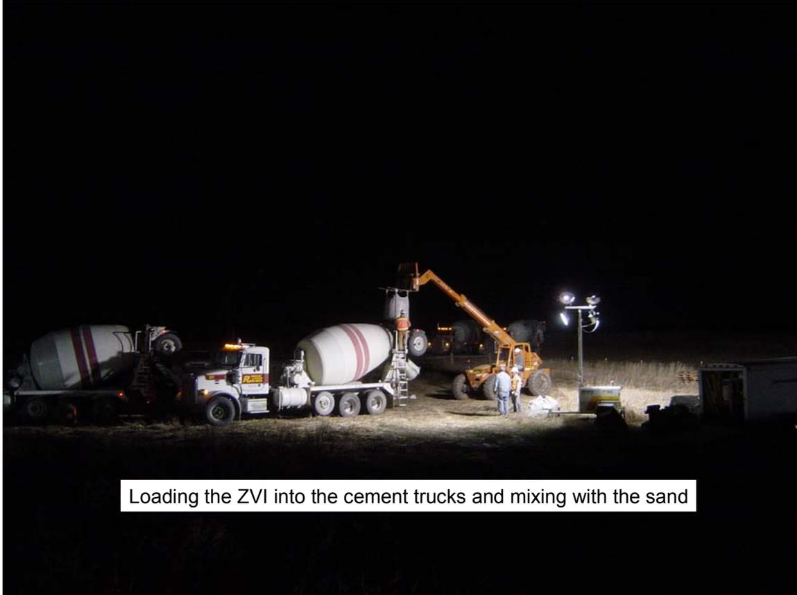
Loading the ZVI into the cement trucks and mixing with the sand
