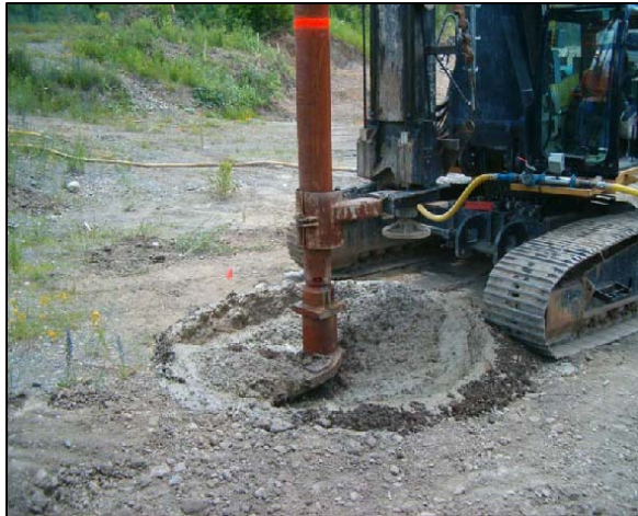
Figure 7-7. In-Situ Soil Mixing at MGP Site
